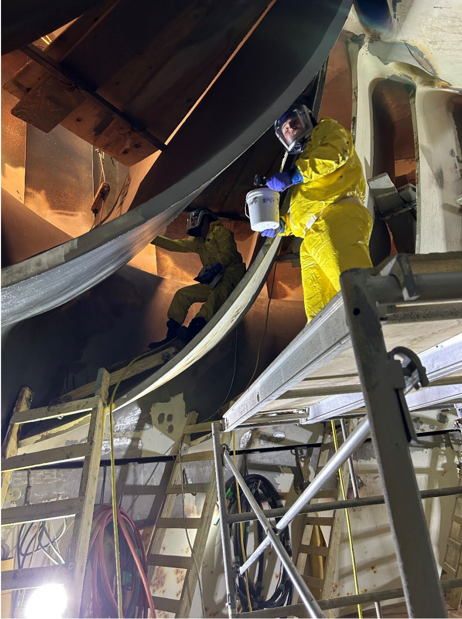
Figure 7.—Application of PE2 to Blade 7.
