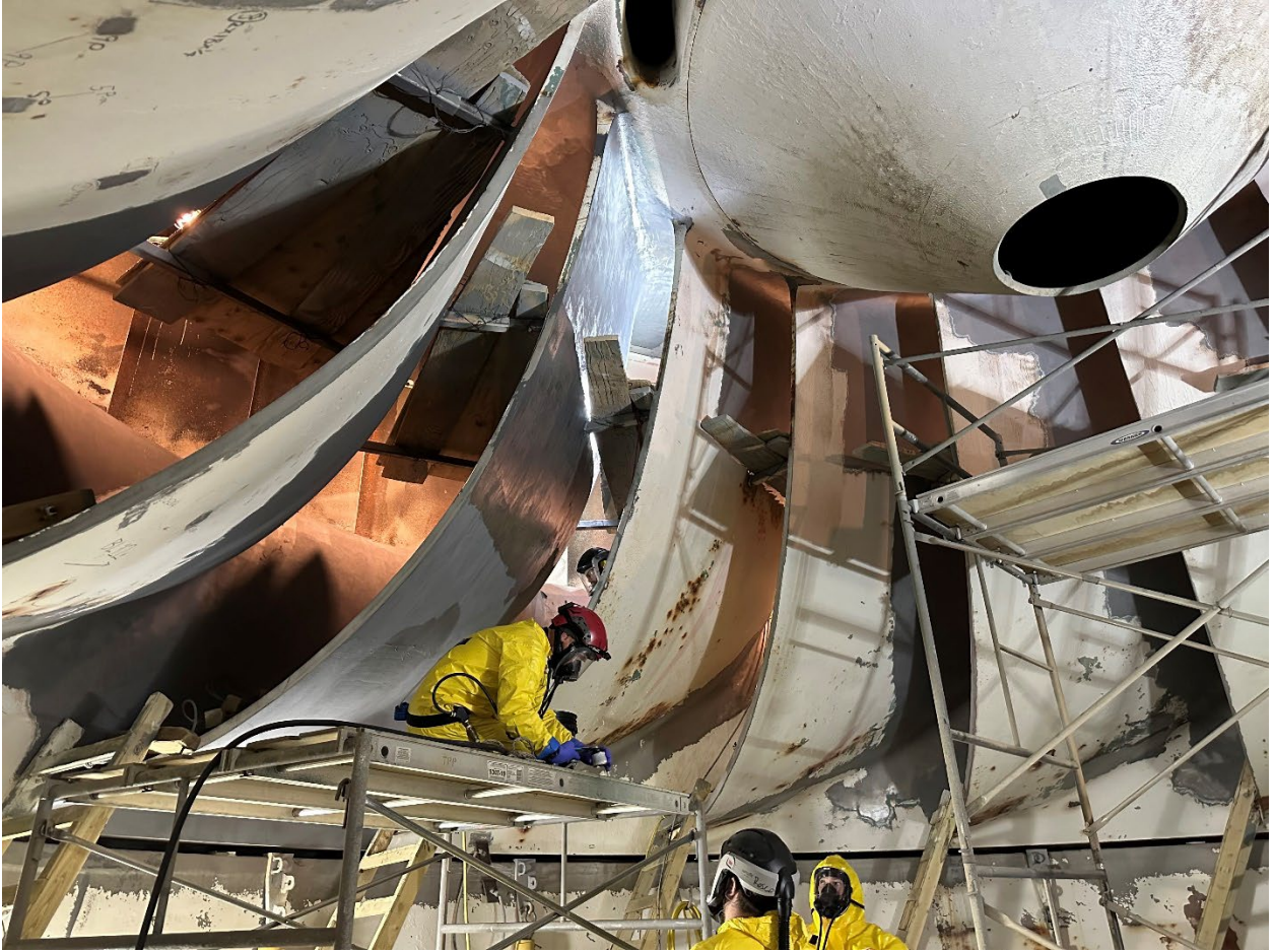
Figure 4.—The team applies adhesive to Blade 13.
